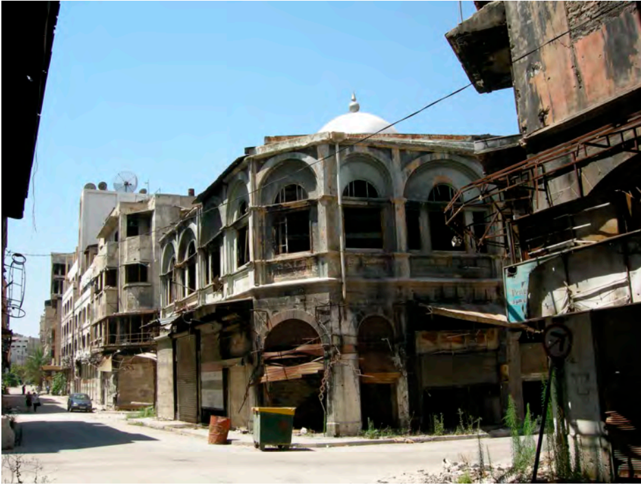
Figure 11.10c Another section of Souk al-Naourah, showing the French-style buildings that used to serve as offices and shops before being destroyed by the recent war. Image: Marwa al-Sabouni
