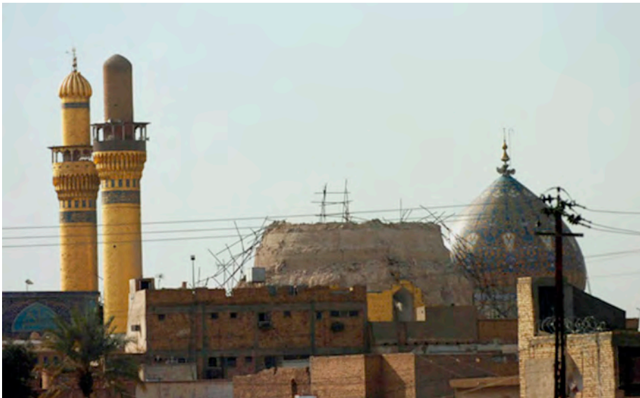
Figure 31.3 The extensive damage to the al-Askari Shrine in Samarra, Iraq in 2006 has been regarded by many as the tipping point that turned general unease with the coalition presence in Iraq into a full-scale, sectarian civil war. The minarets were destroyed in 2007. Image: PJF Military Collection / Alamy Stock Photo
