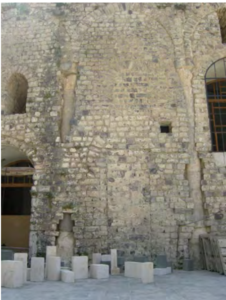
Figures 11.6b–c The war inflicted great structural damages to the mosque, revealing older pillars from a previous structure buried within its walls. These remnants might be seen as indicative of a unique preservation approach that opted not to tear down, but rather to build on. Image: Marwa al-Sabouni
