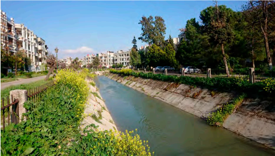
Figure 11.9a A 2021 photo of the irrigation network running through the city. Municipal decisions to let the water flow are followed by others to restrict it, an on-and-off approach not explained to the public. Image: Marwa al-Sabouni
