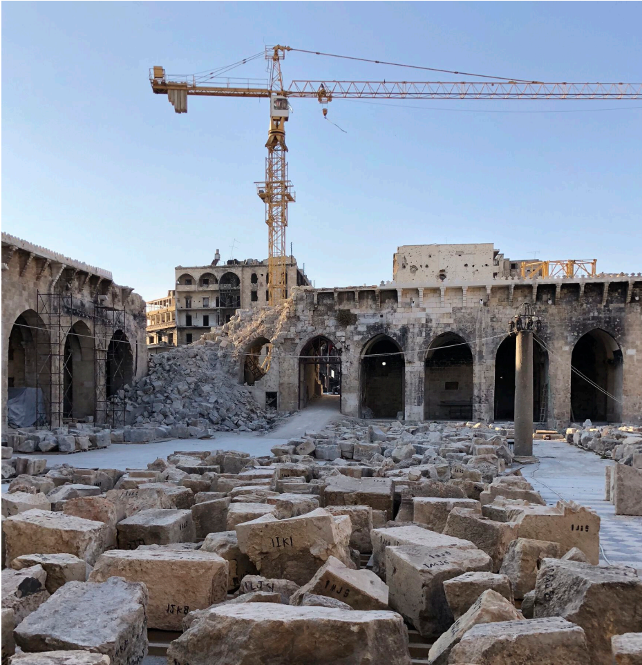
Figure 10.6 Damage to the Great Umayyad Mosque of Aleppo, including damage to the minaret. Image: Francesco Bandarin
